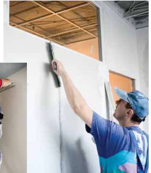
Plastering the board joints in partitions (left) and the junctions of wall and ceiling (above).
