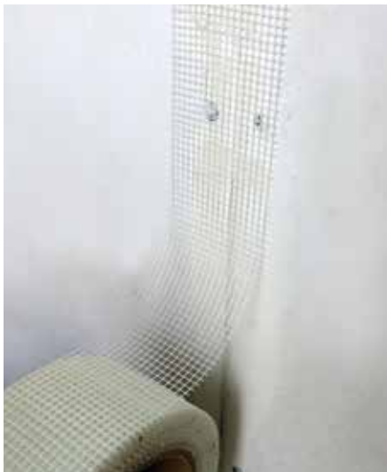
Fill joint with single, thin layer of plaster and then overlay reinforcing mesh.
