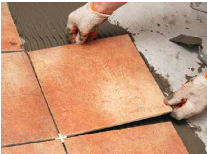
Applying tile adhesive on any SUPALUX® boards prior to tiling.
