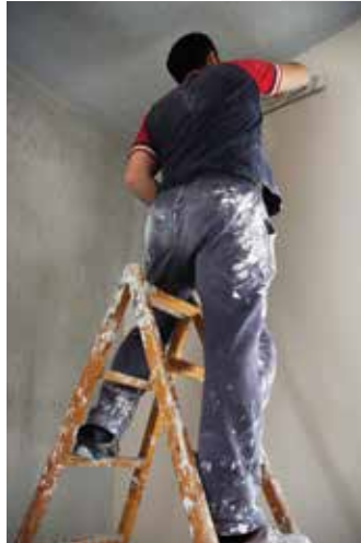
Plastering the board joints in partitions (left) and the junctions of wall and ceiling (above).
