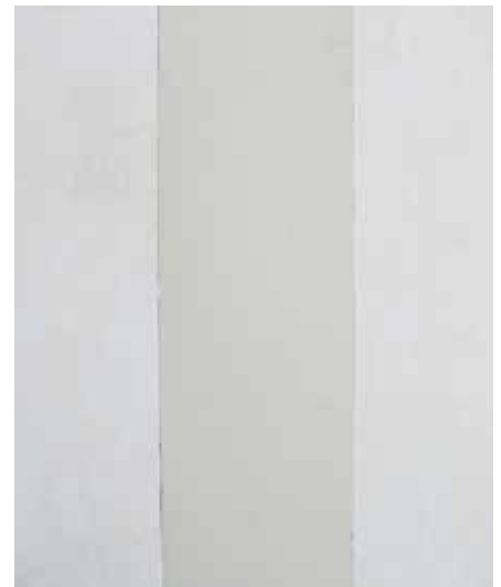
Final joint after finishing with trowel.
